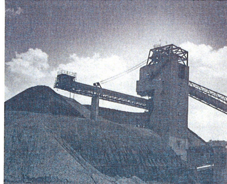
coal stacker tower & coal pile
