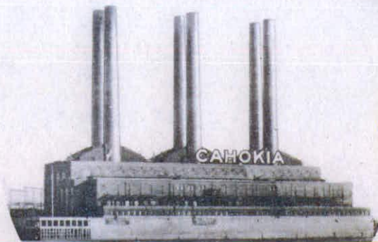
Cahokia Power Plant
