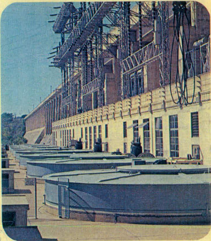
Outside view of "main deck" of power station. The circular covers protect the generators from the weather.
